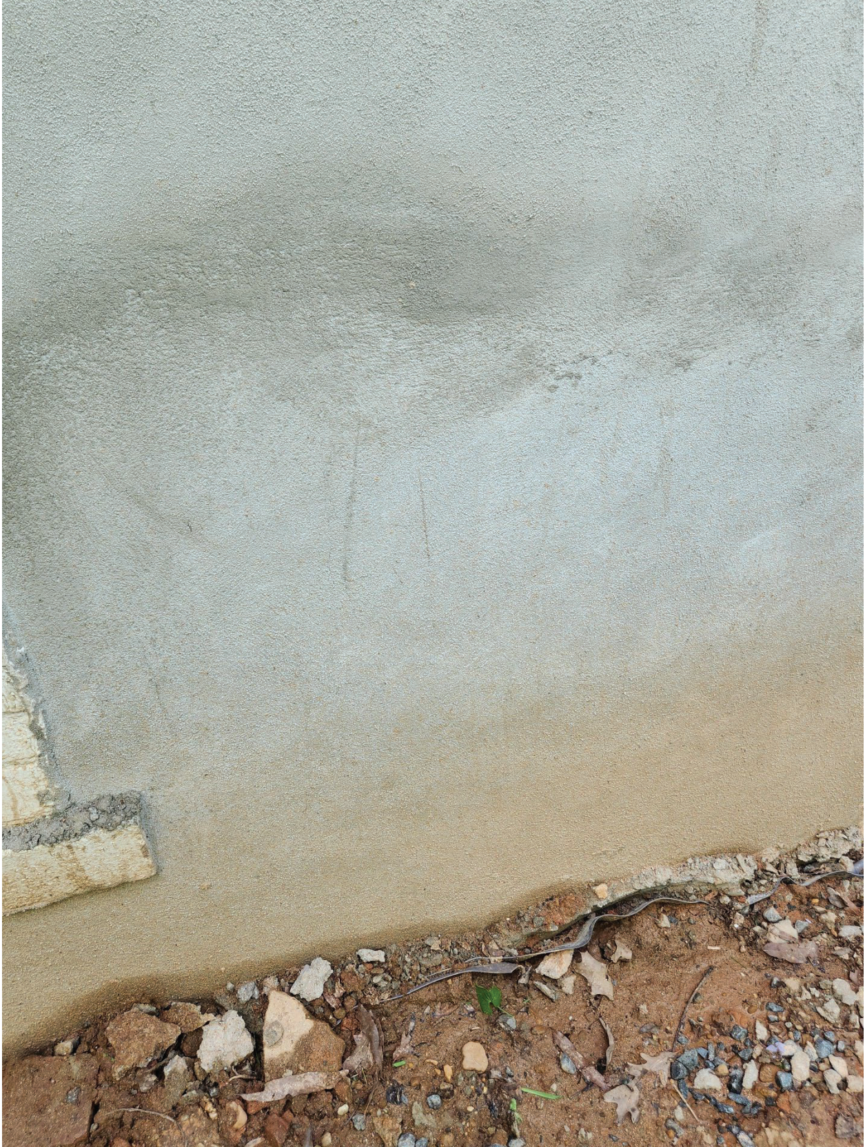
Example of finish of walkway
