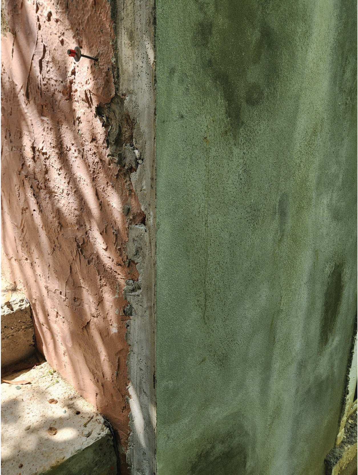
Example of finish of walkway
