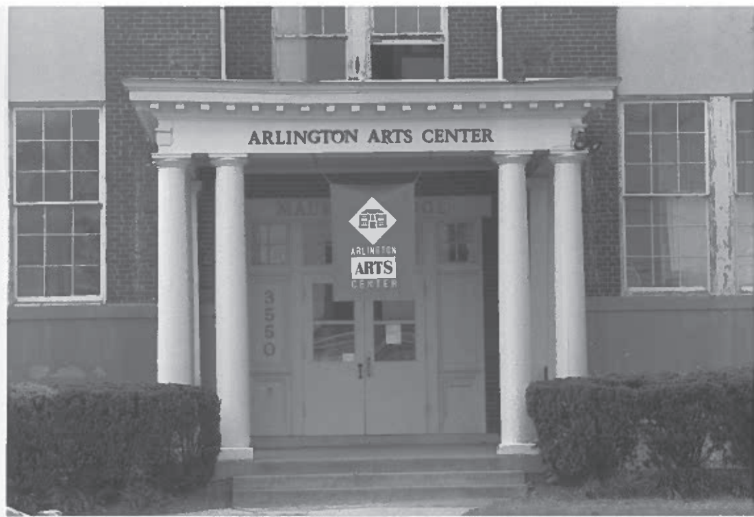
Banner on building in 1990s
