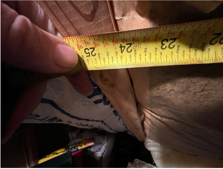
Figure 10: Spacing between 2 Rafters is 24" inch on center.
