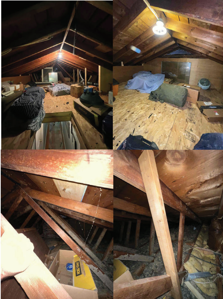
Roof Structure From Attic
