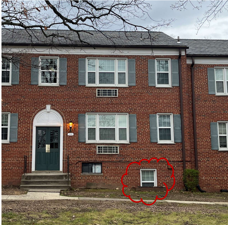
EXISTING WINDOW WELL AT BUILDING 16
