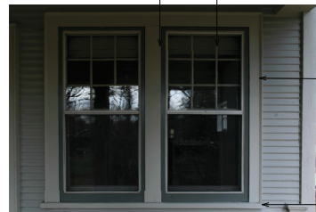
PROPOSED WINDOWS TO MATCH EXISTING MUNTIN PROFILE AND BE INTEGRAL TO GLASS PANES
