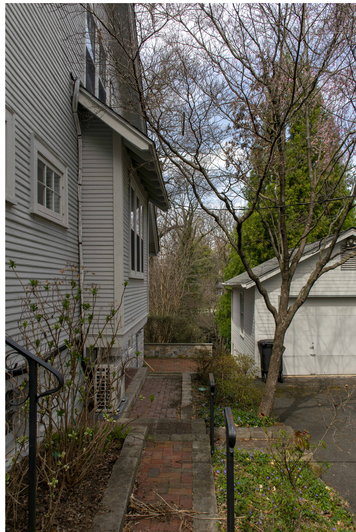
BRICK PAVER TO BE REPAIRED AS NEEDED IN AREAS WHERE DESIGNATED TO REMAIN
