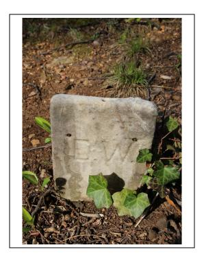
Marker Notes: Marker has one weep hole at the top and two weep holes in the face
