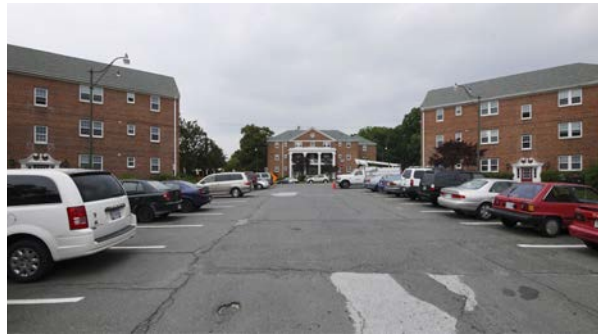
Existing Conditions, Arbor Heights Apartments
