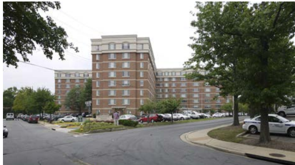
Existing Conditions, Dominion Plaza Apartments
