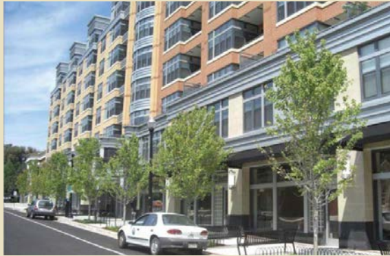
Mixed-Use Buildings Variety of Scales
