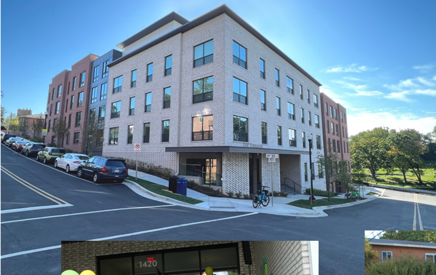
Arlington View Terrace – East (Completed)
