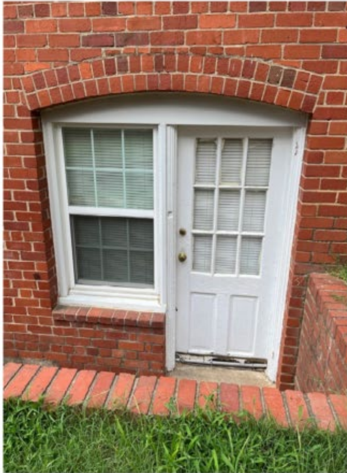
/ BUILDING 30 EXISTING REAR ENTRY DOORS
