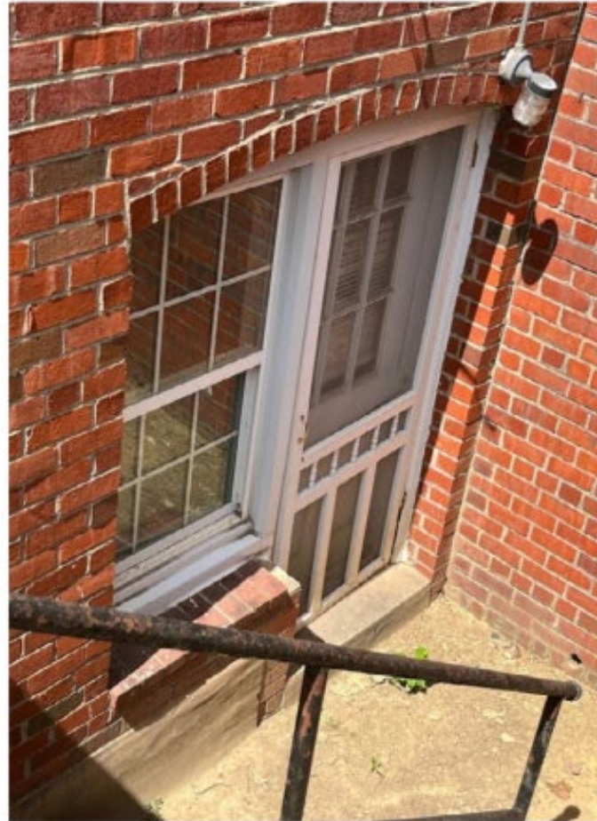
/ BUILDING 32 EXISTING REAR ENTRY DOORS
