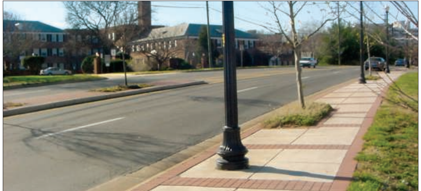
Improved sidewalks and new medians enhance both the aesthetics and safety of the Pike for pedestrians, bicyclists and motorists alike.
