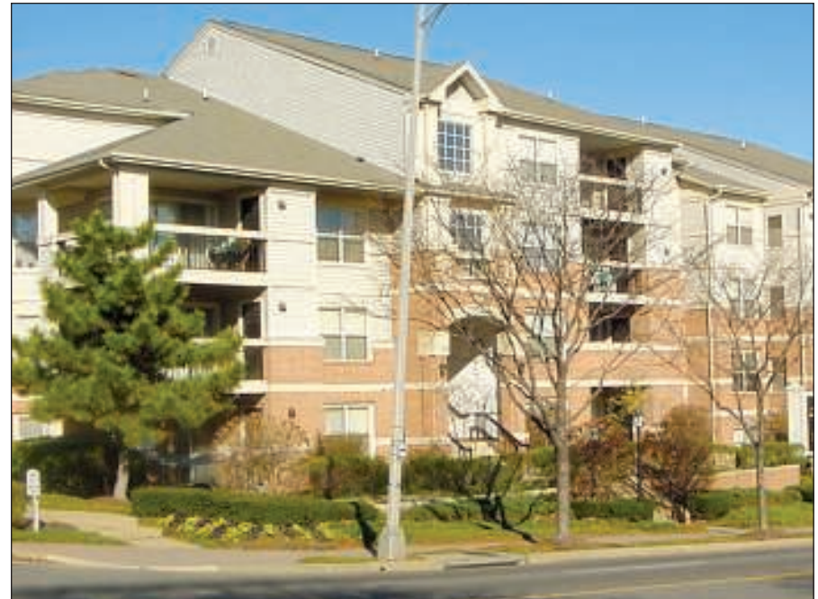
Newer multifamily housing along the eastern end of the Pike is a sign that interest in this area is building within the development community.
