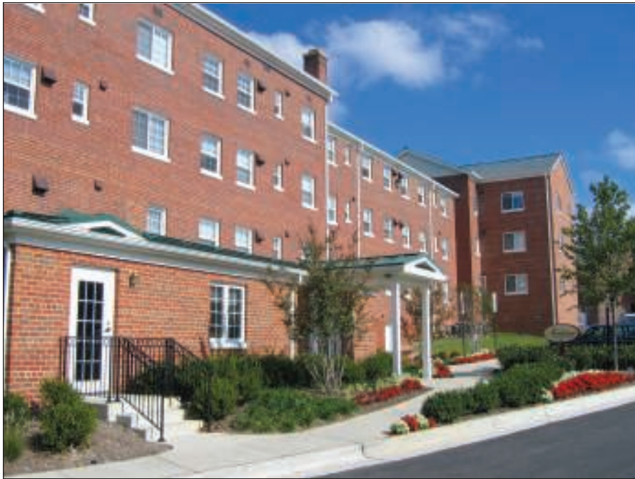
The Monterey/Sierra redevelopment project preserved 96 affordable rental units, while creating new homeownership opportunities in the Columbia Heights West neighborhood.
