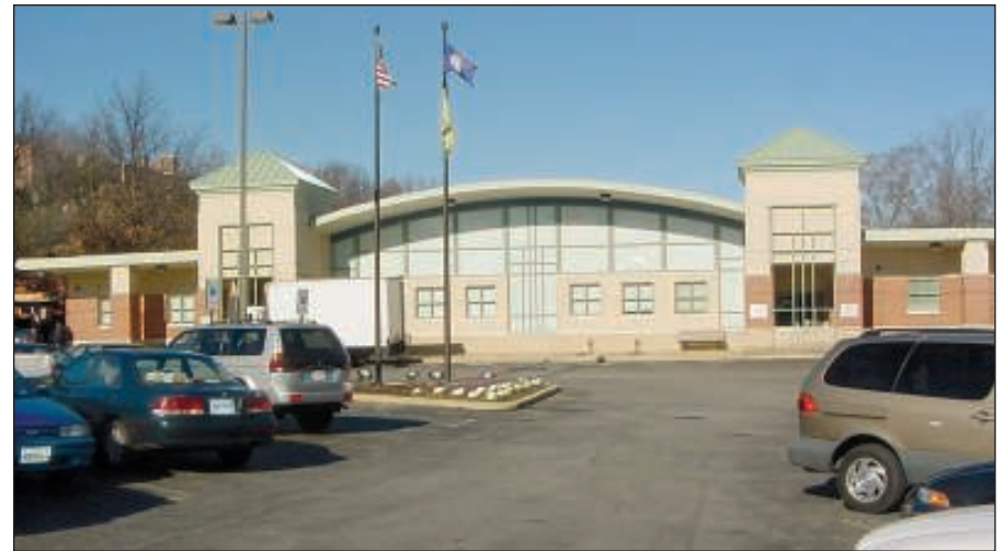
Construction of a new Arlington Mill Community Center is slated to begin in 2007.
