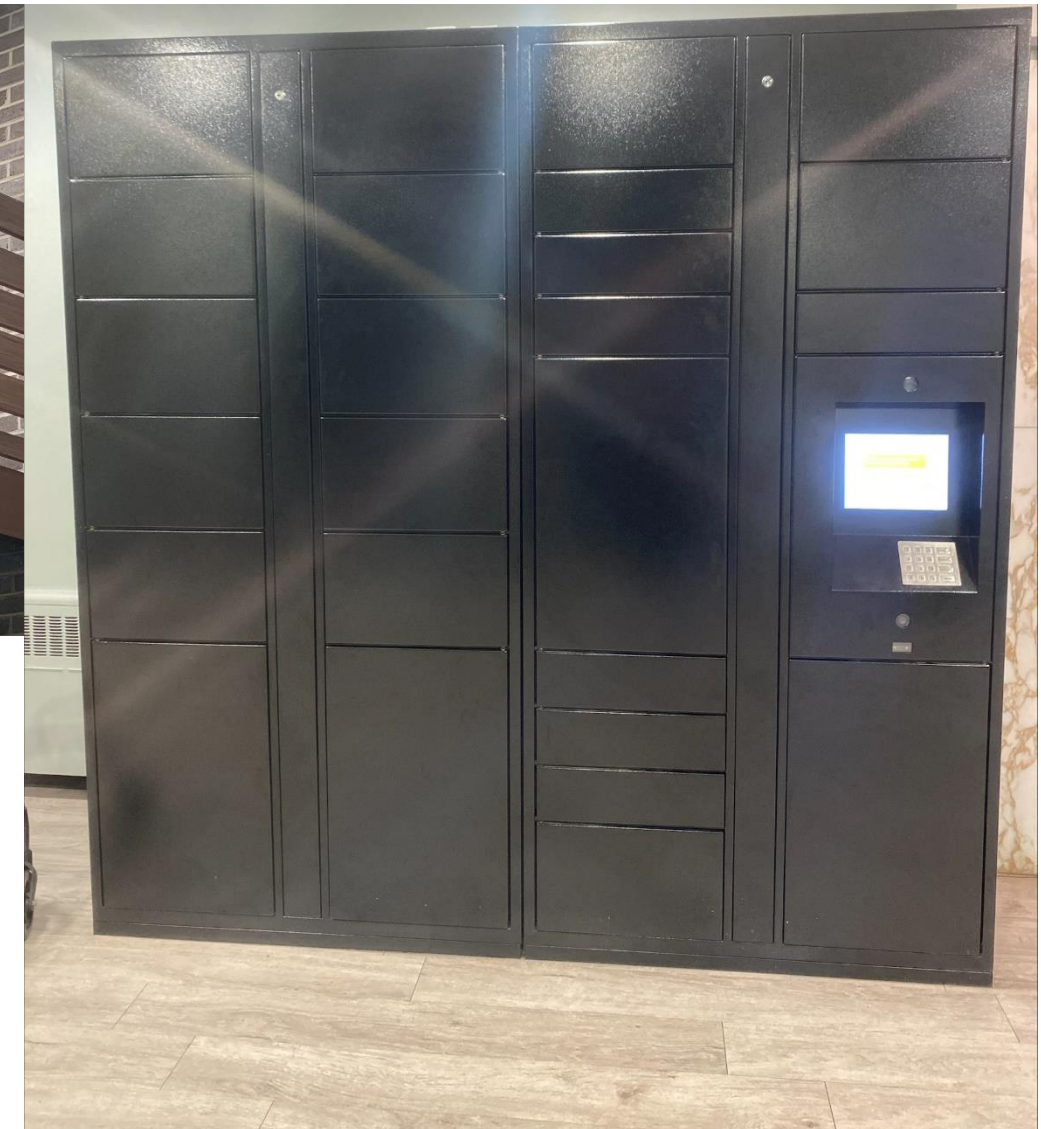
Lockers installed for packages
