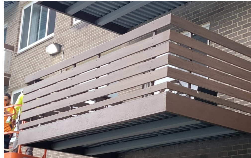
Completed all balcony repairs
