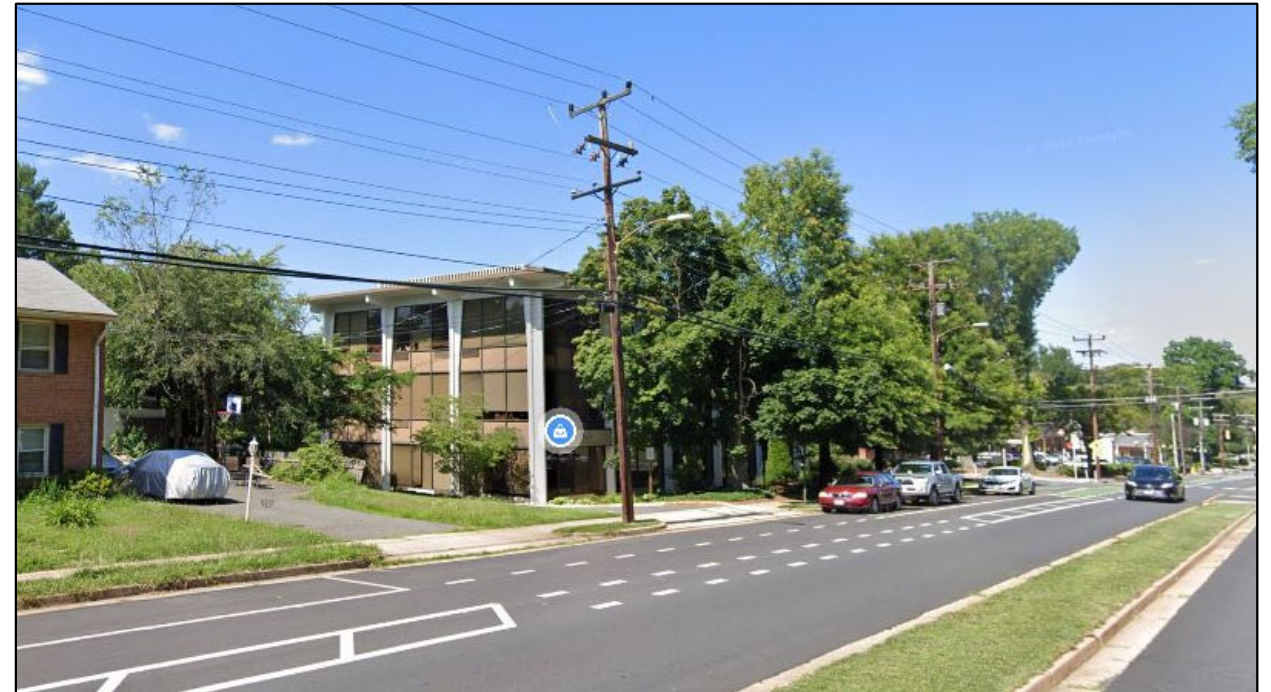
Current site development.
