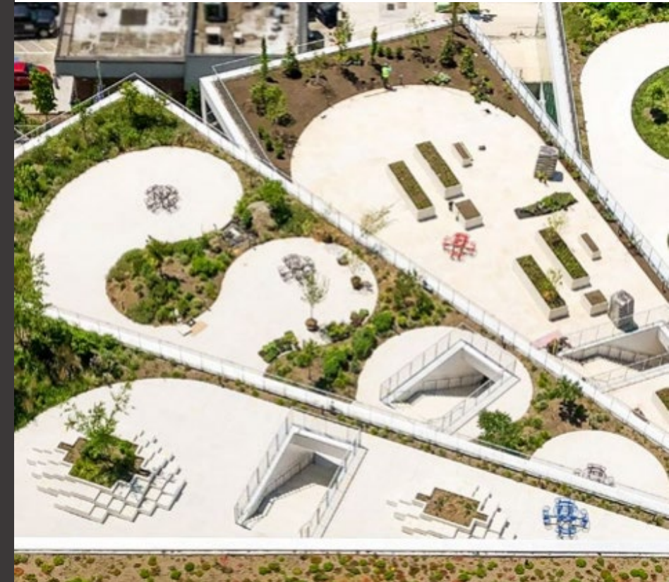
Green roof with trees at APS's Heights Building
