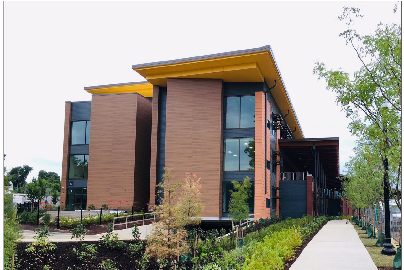
Alice West Fleet Elementary – Completed in 2019
