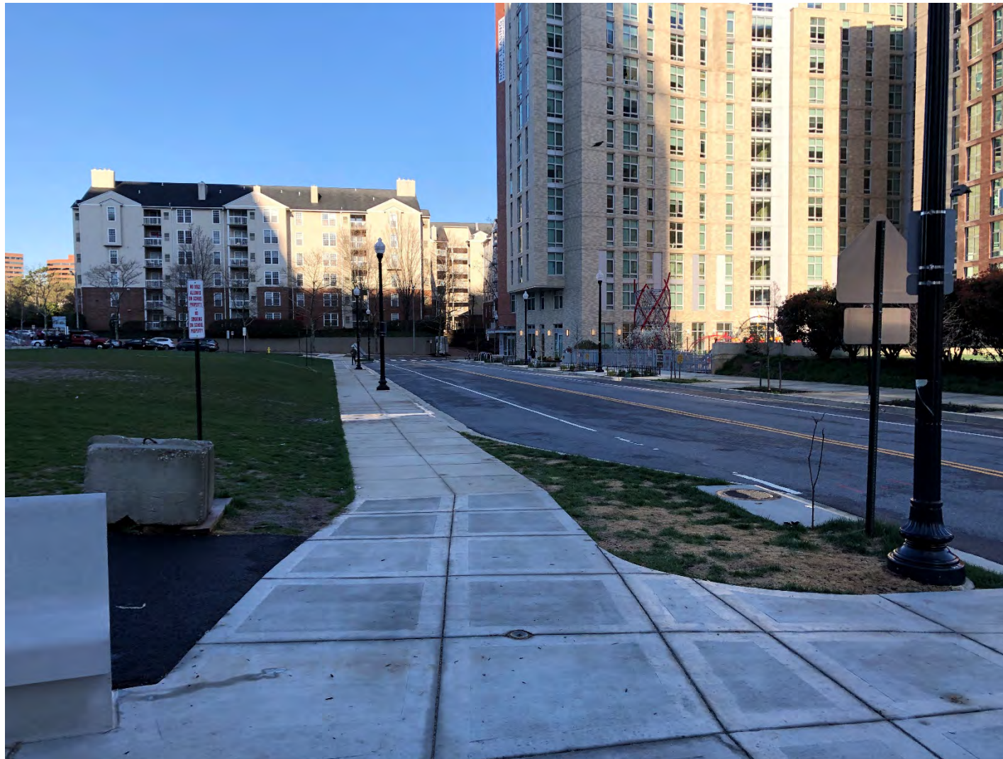
18th St N at Rosslyn Highland Park Looking West Toward N Quinn St
