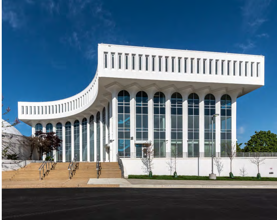
Precedent: KEIM coating applied at the recently completed APS Education Center Reuse project.
