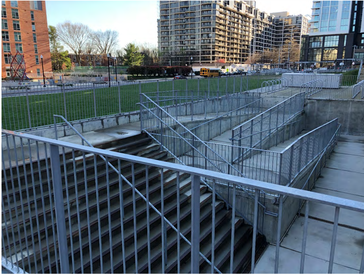
Temporary Stair and Ramp to Heights Building G1 Level (Shriver Administrative Area)
