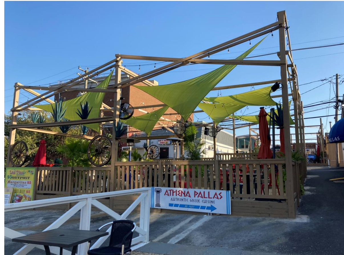
TOSA w/ affixed canopy & railing
