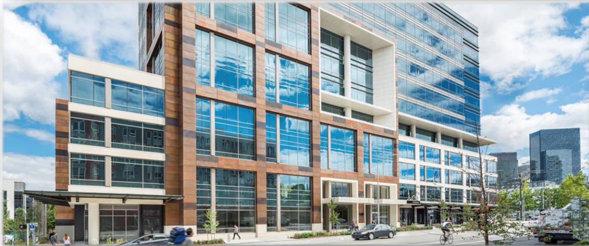
400 Dexter Biotech Office Building, 298,000 sqft, South Lake Union, Seattle, WA
