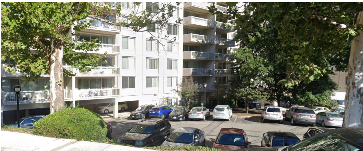
Figure 5b: View of Crystal Towers near the Intersection of 18 th Street S. and S. Fern Street
