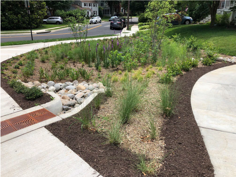
A "green street" on Larrimore St
