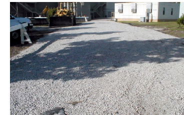
Install stone construction entrance on driveway to be removed
