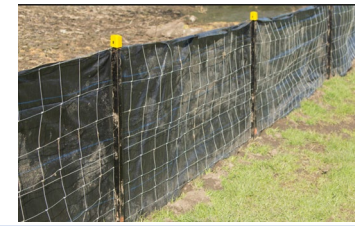
Install temporary silt fence during construction along the disturbed area
