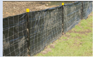
Install temporary silt fence during construction along the disturbed area
