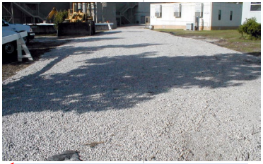
Install stone construction entrance
