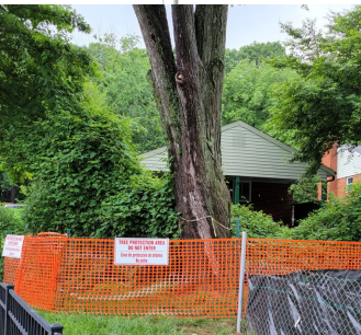
Install tree protection
