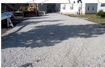
Install stone construction entrance
