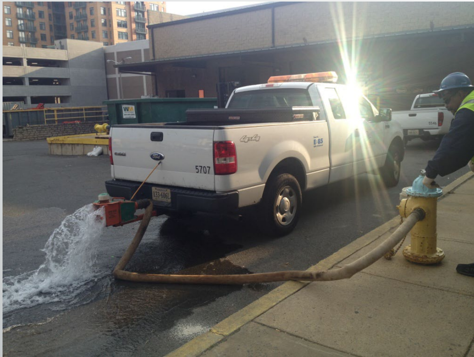
LPD-250 Diffuser – NOT attached directly to the Fire Hydrant
