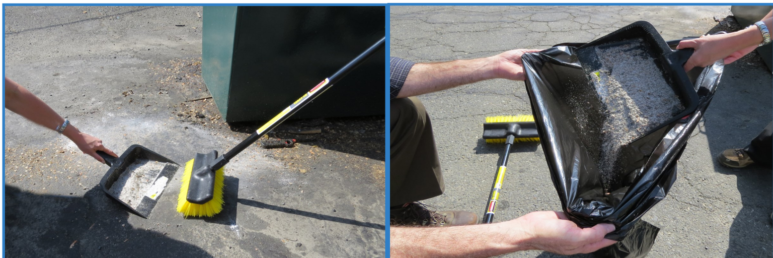
Sweep up the absorbent material and grease, bag it, and dispose of it in the trash.
