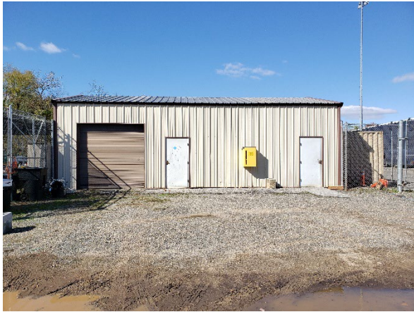
Photo 1: Maintenance Building with mounted spill kit
