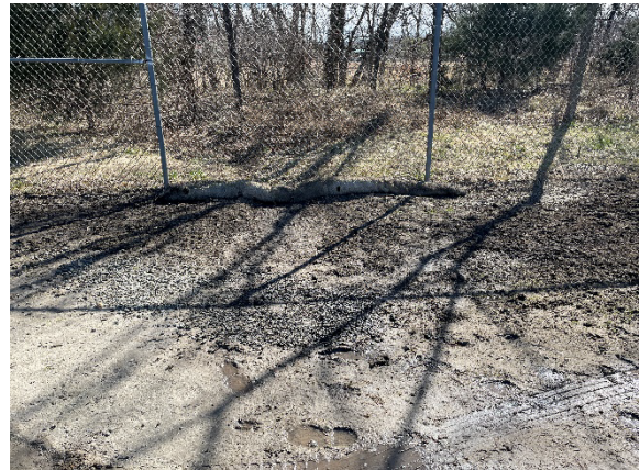
Photo 6: Boom and stone berm at east drainage low spot
