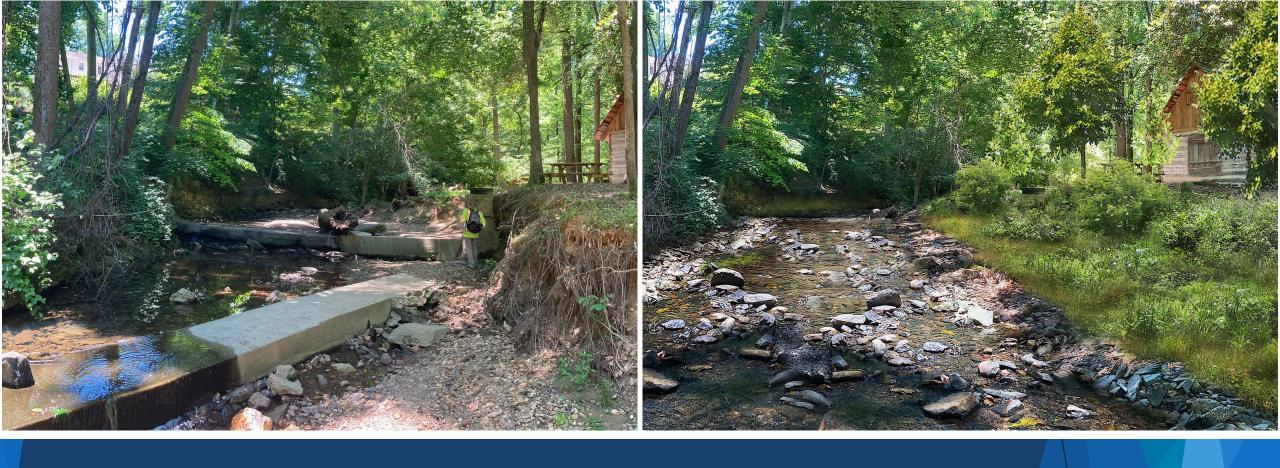
Raise Stream Bed, Re-Bury Sanitary Sewer Pipes, Stabilize Stream Channel
