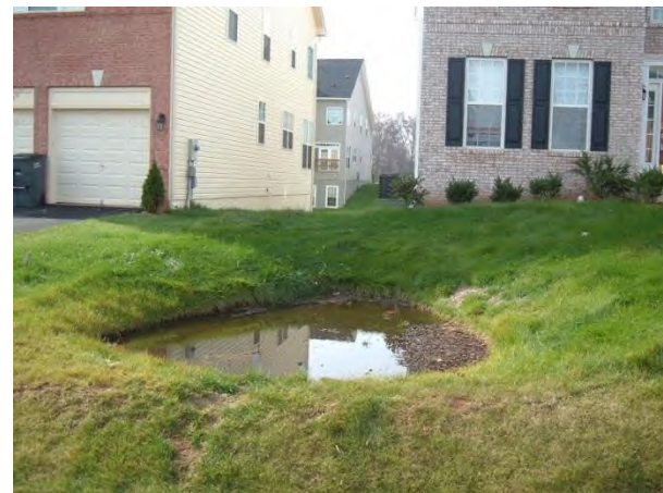
Examples of failed rain gardens
