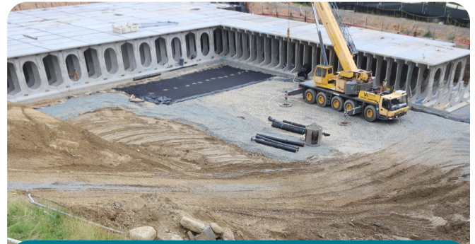
Figure 1 - Cardinal School storage under construction
