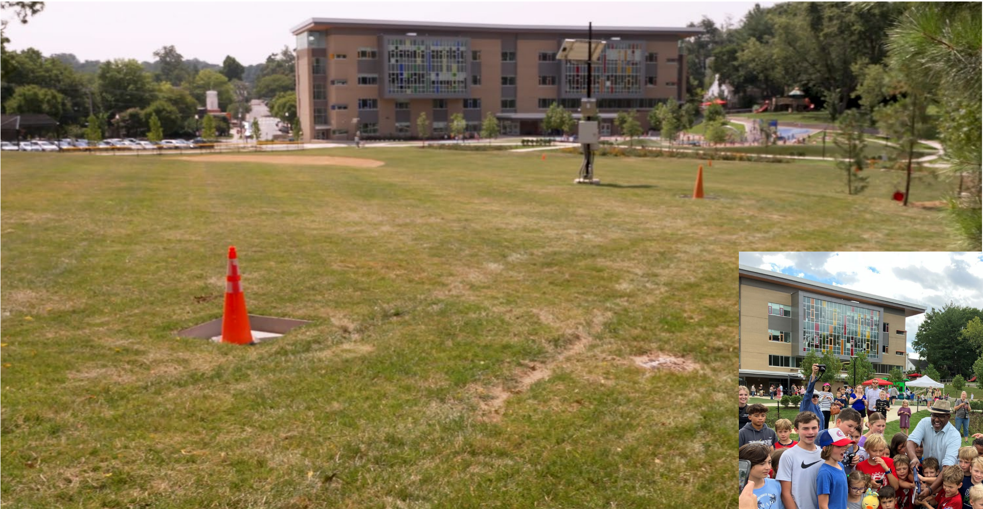
Fields over the Stormwater Vault at Cardinal School. Cones mark access ports, which will have artificial turf installed over them. A community-initiated celebration occurred on September 30.
