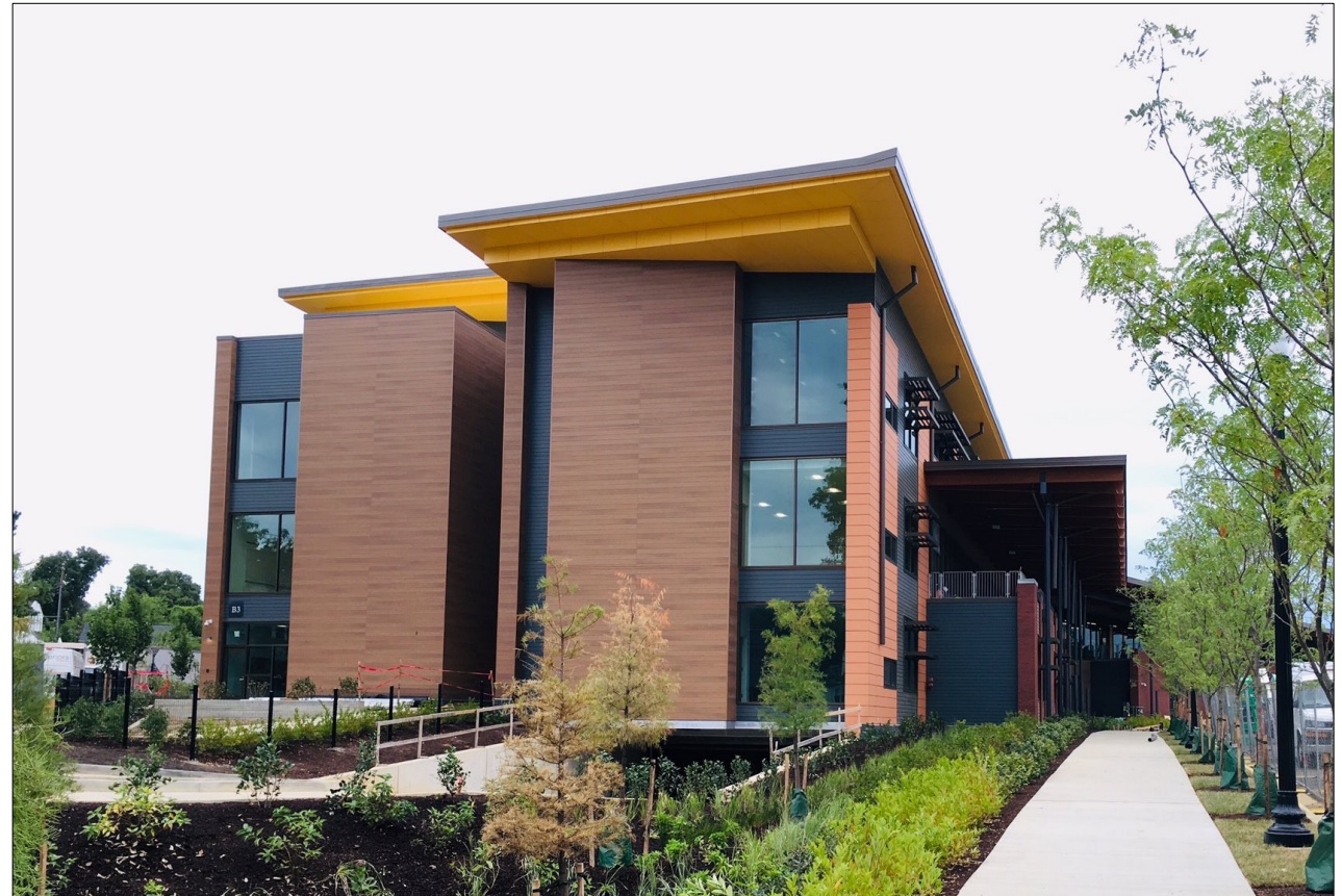
Alice West Fleet Elementary – Completed in 2019
