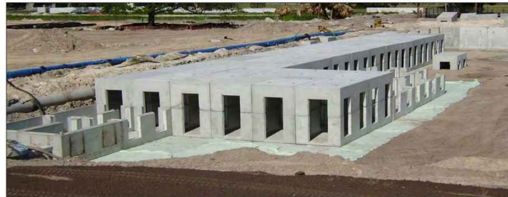
StormCapture System During Installation Process
