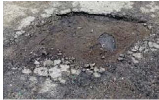
Paving Program - $128 M
