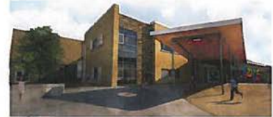
Discovery Elementary School: Completion September 2015 New net zero energy school providing 630 seats
