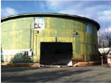
Existing 26 th St. Salt Dome
