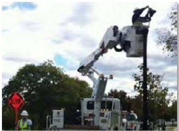
Street Light Maintenance Crew at Work
