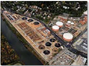
Aerial View of Arlington's WPCP
