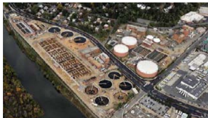
Water Pollution Control Plant - $86.7 M
