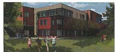
McKinley Elementary School: Completion September 2016 27,000 sq. ft. addition, plus renovation providing 241 new seats.
