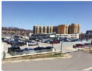
Trades Center Parking Garage
