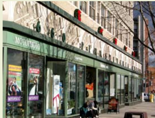
660 Pennsylvania Ave. SE, Washington, DC
