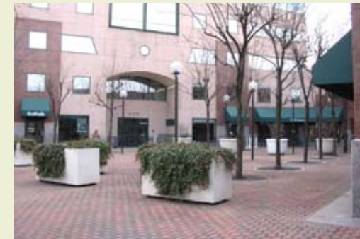
Plaza at the Olmsted Building
