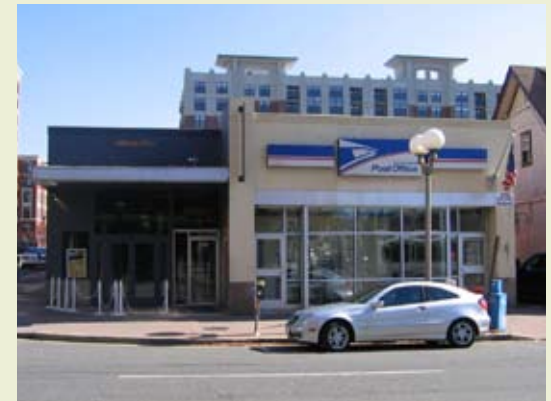
1041 North Highland Street
