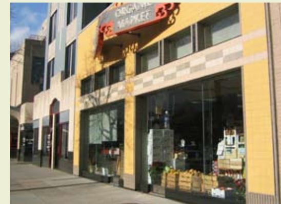
648 Pennsylvania Ave. SE, Washington, DC
