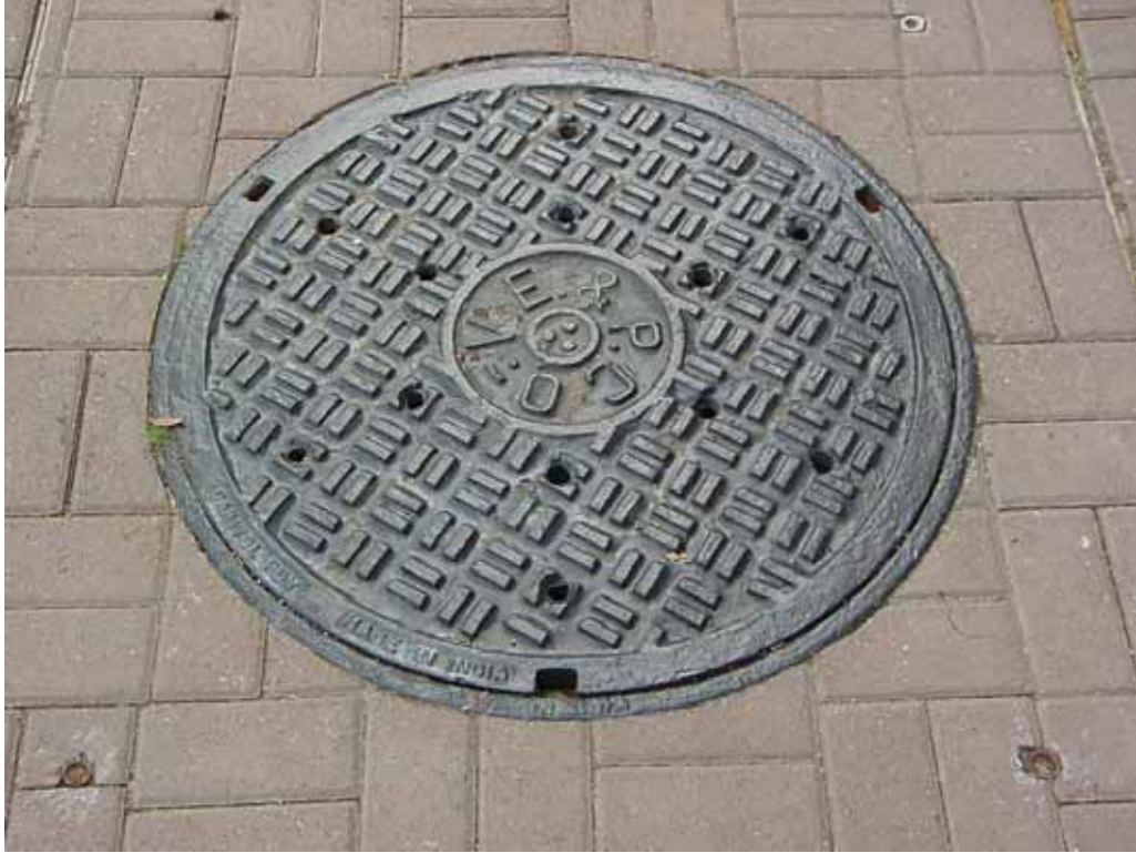
FIGURE 15. Installation of Manhole Cover
