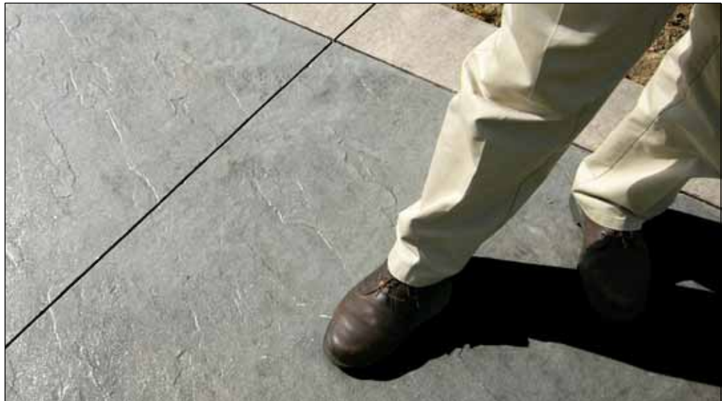
FIGURE 2. Example of Acceptable Clear Zone Treatment (slate texture) Detail of slate texture. Note the directional pattern.
