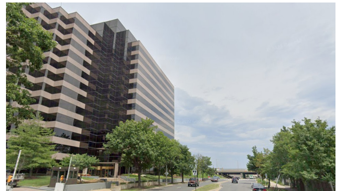
⑥ S FERN ST LOOKING NORTH
