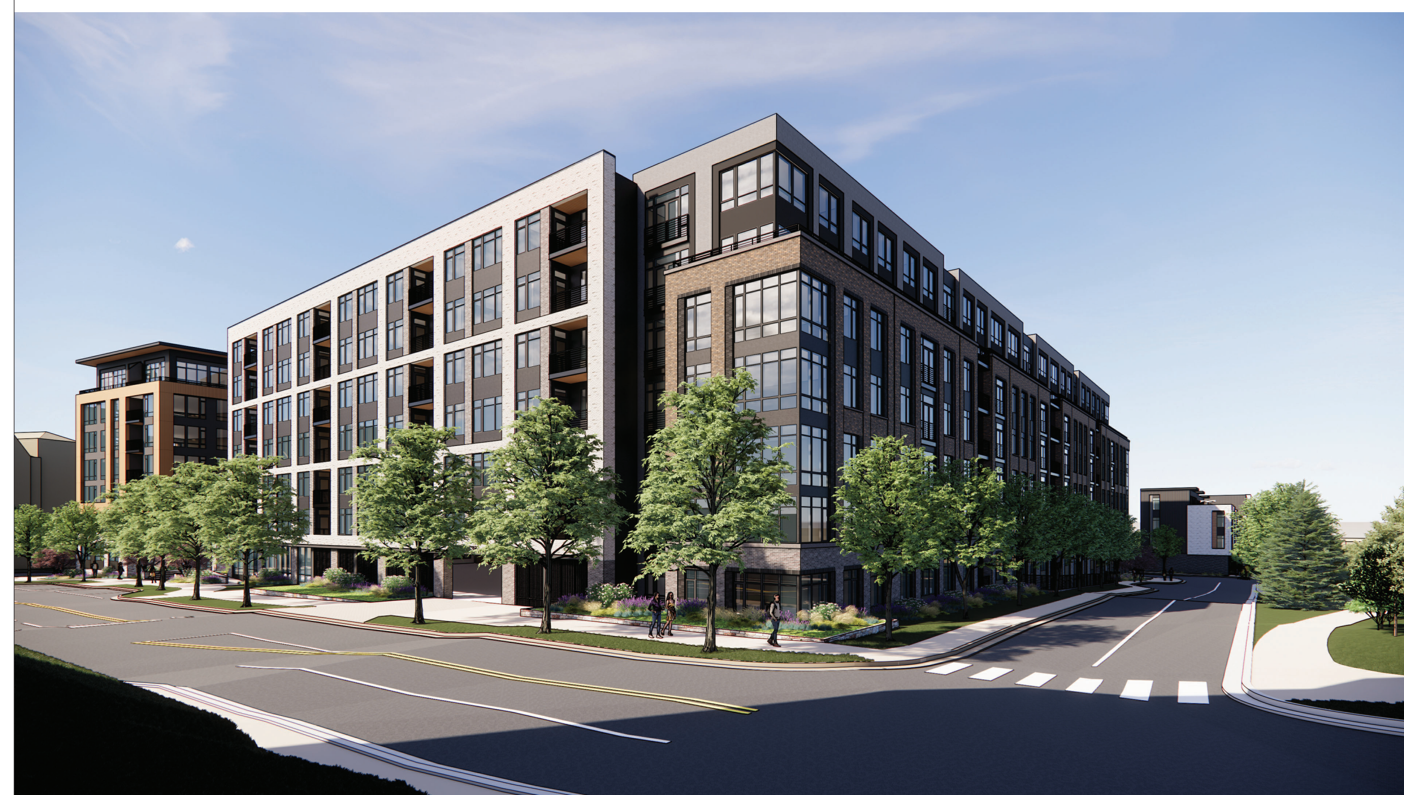
3 --- BLDG E - NORTHWEST VIEW
