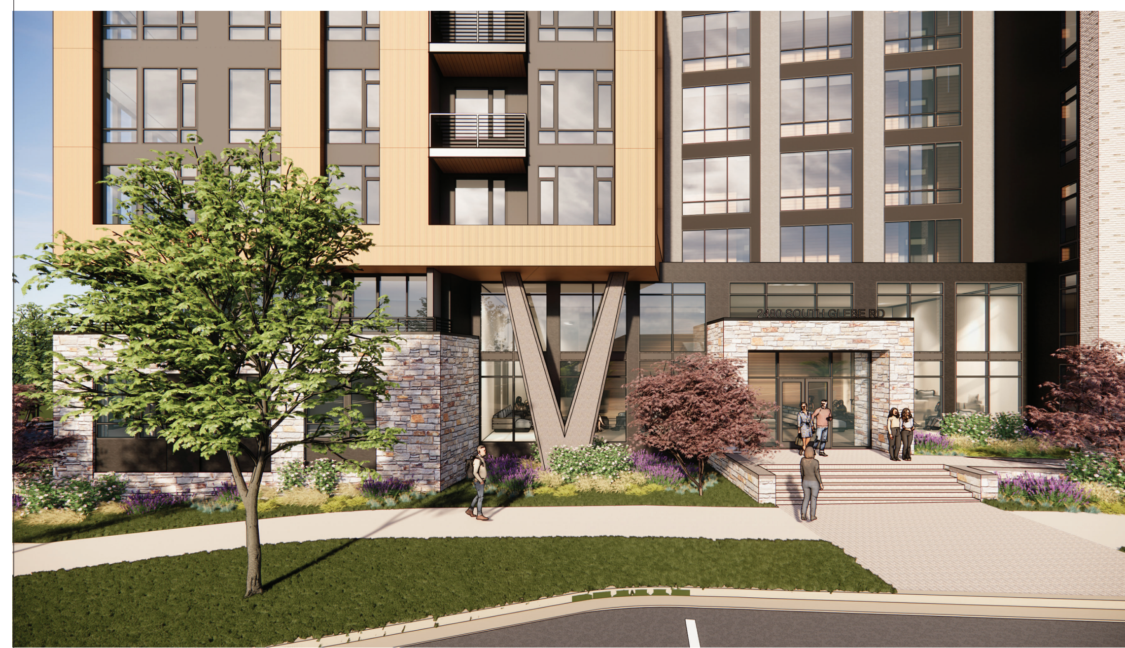
3 --- BLDG E - MAIN ENTRY CLOSEUP
