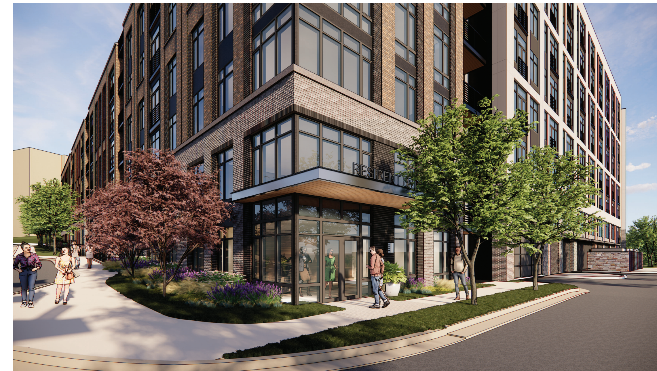
2 --- BLDG E - SECONDARY ENTRANCE OFF PRIVATE DRIVE
