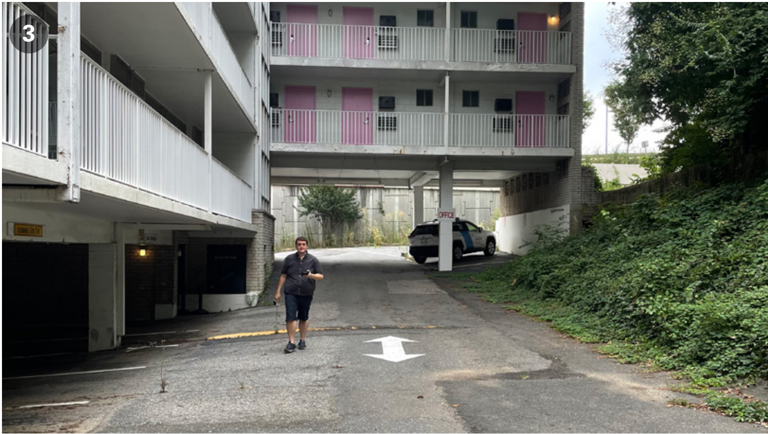
VIEW FROM WEST
