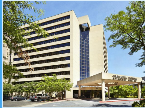
Embassy Suites Hotel 1393 S Eads St
