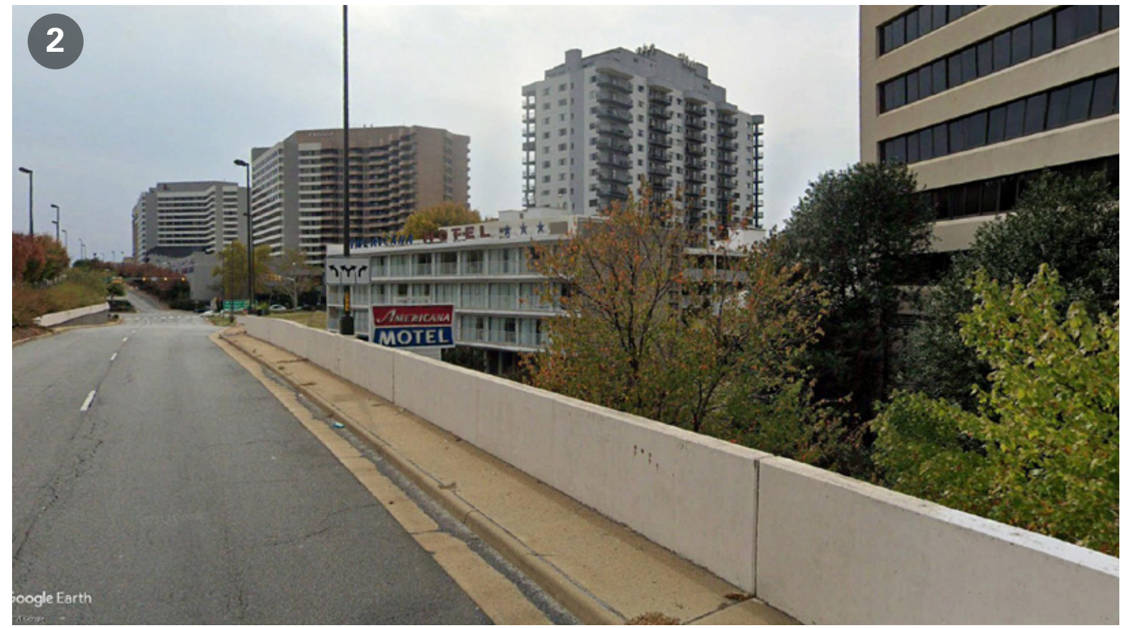
VIEW FROM NORTHEAST
