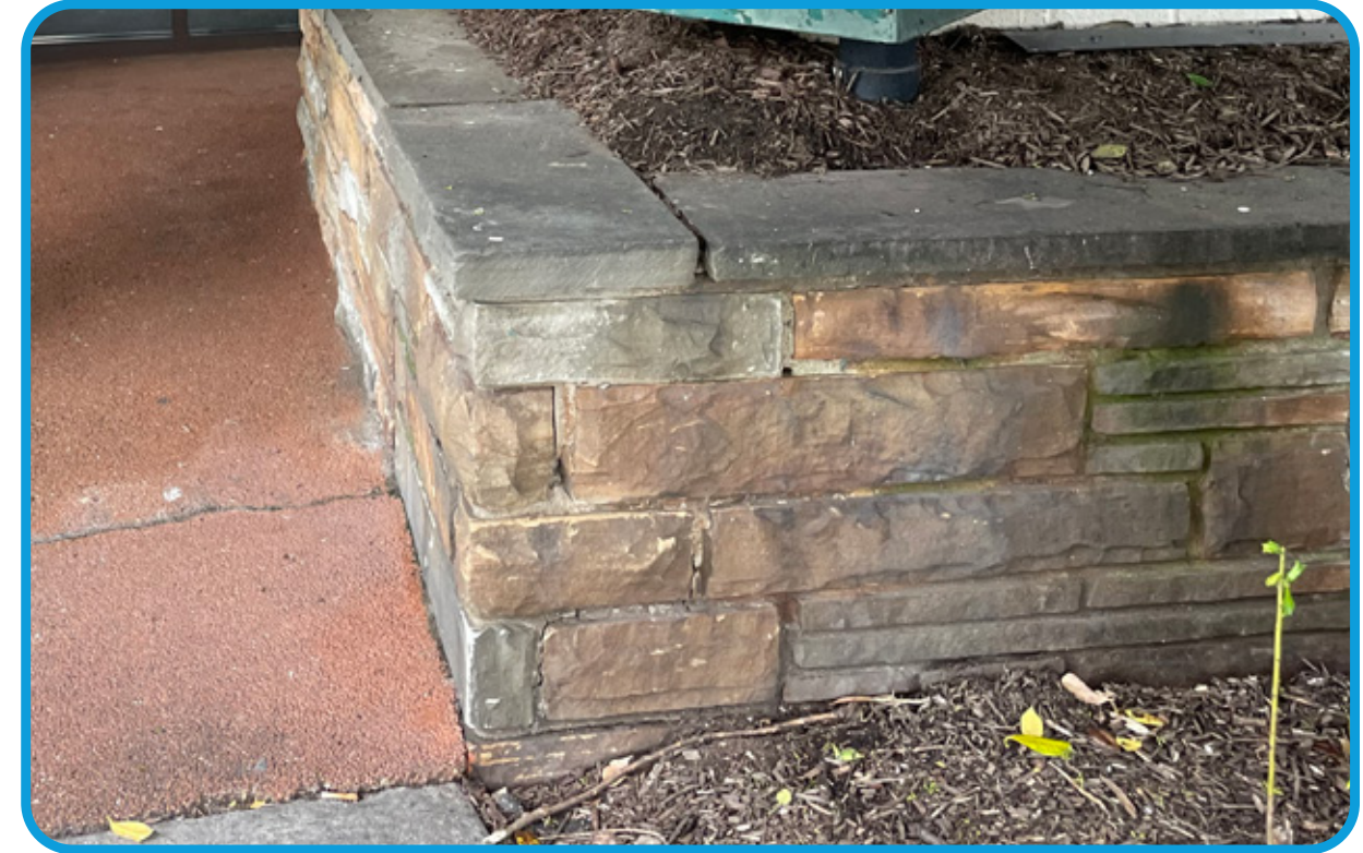
STONE BASE MATERIAL (REUSE OR REPLACE-IN KIND)
