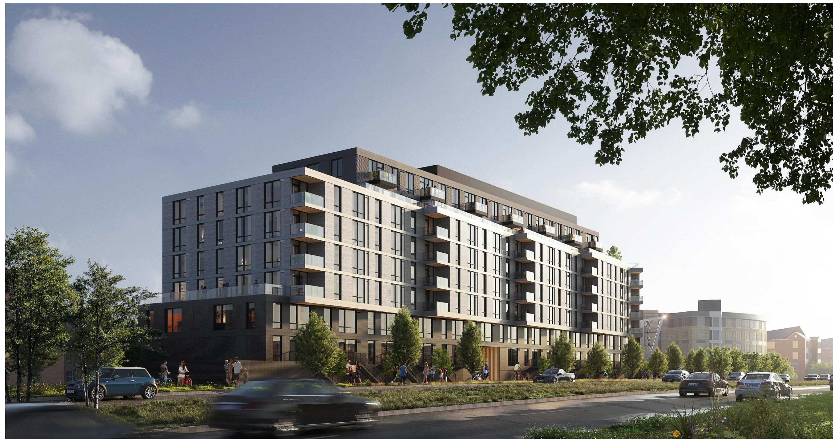
1 CONTEXT VIEW - ARLINGTON BLVD NORTHBOUND - LOOKING NORTH N.T.S
