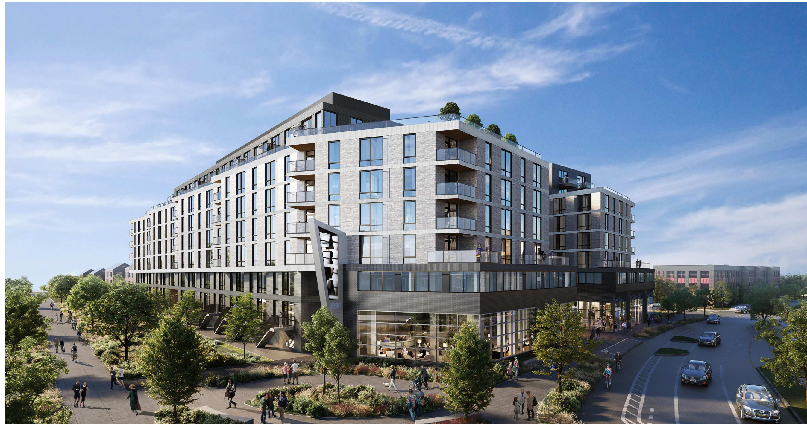
4 CONTEXT VIEW - ARLINGTON BLVD & PERSHING DRIVE - LOOKING SOUTH WEST N.T.S
