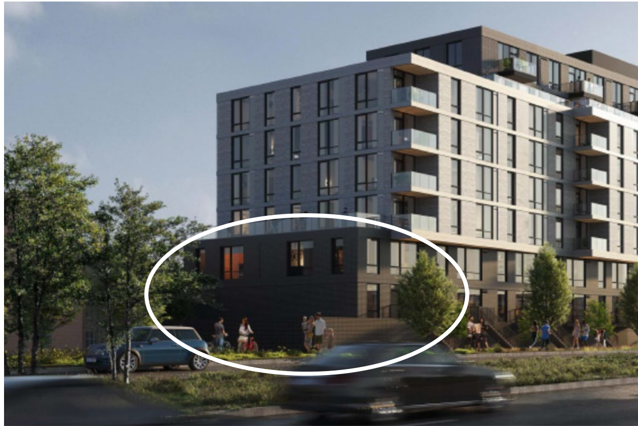
1 | CONTEXT VIEW - ARLINGTON BLVD NORTHBOUND - LOOKING NORTH NTS
