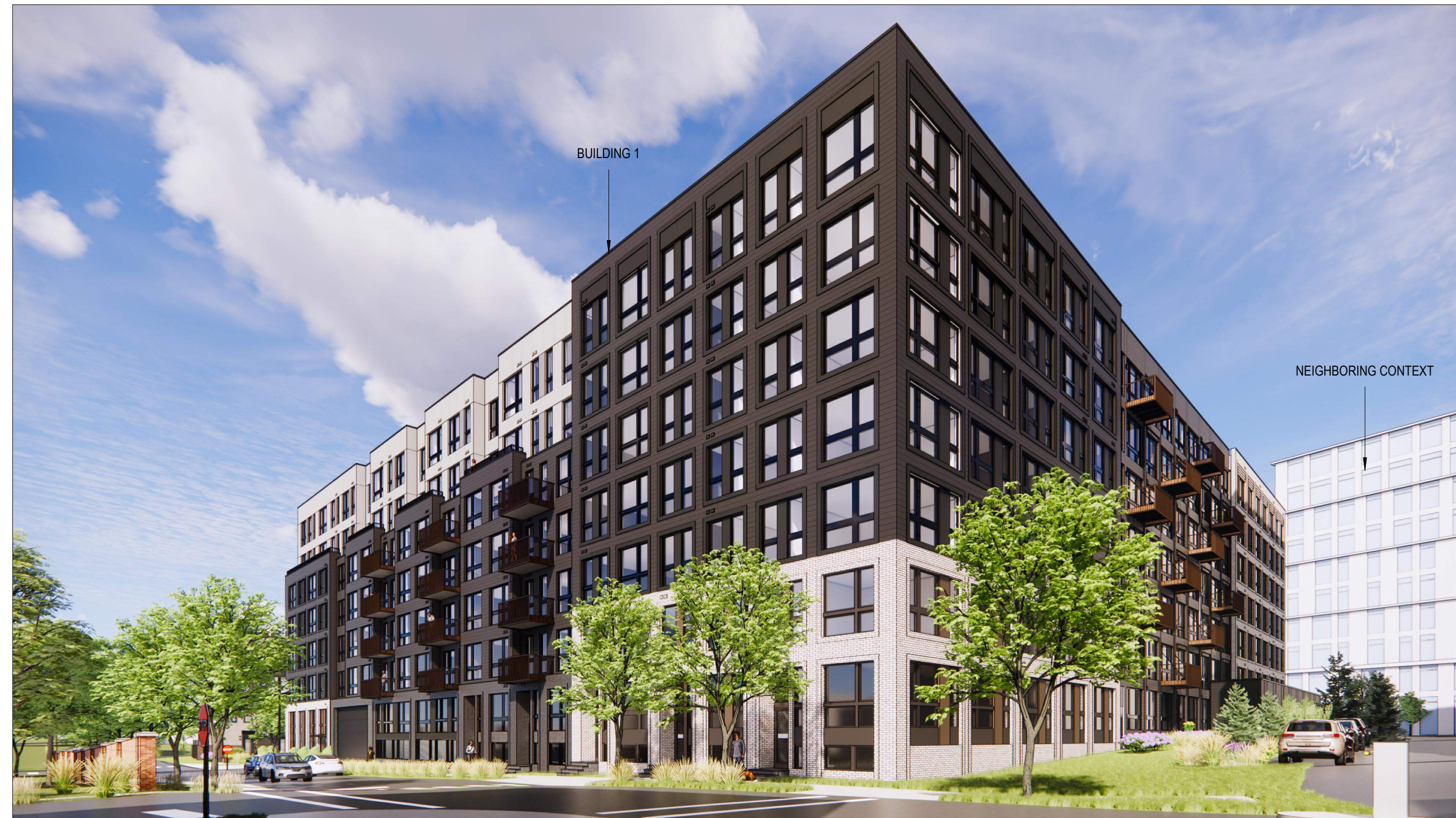
3 - BUILDING 1 SE CORNER
