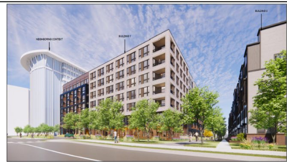
2 - BUILDING 1 NW CORNER
