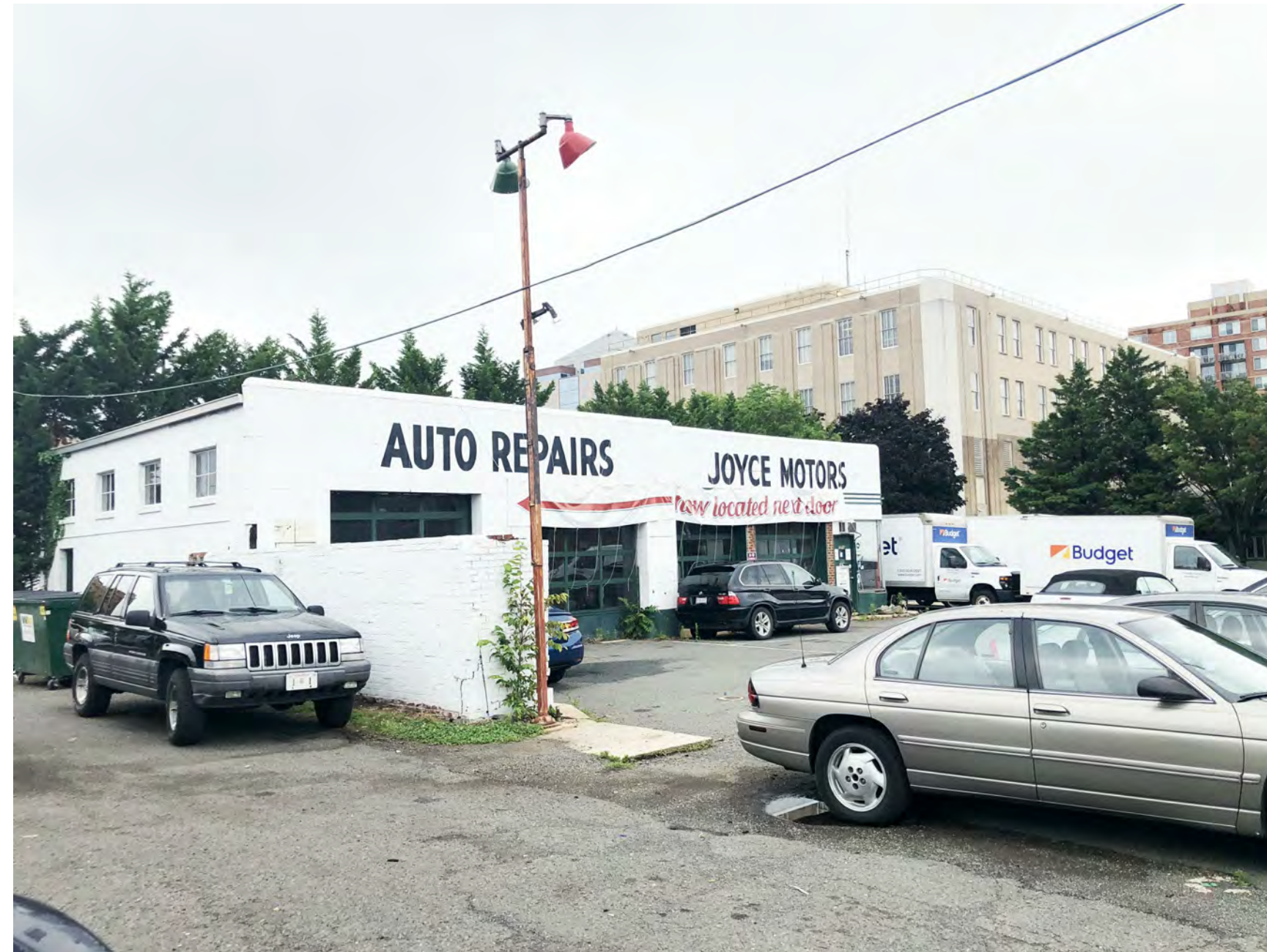
8) VIEW FROM THE EXISTING ALLEY LOOKING NORTHEAST AT THE JOYCE MOTORS BUILDING.
