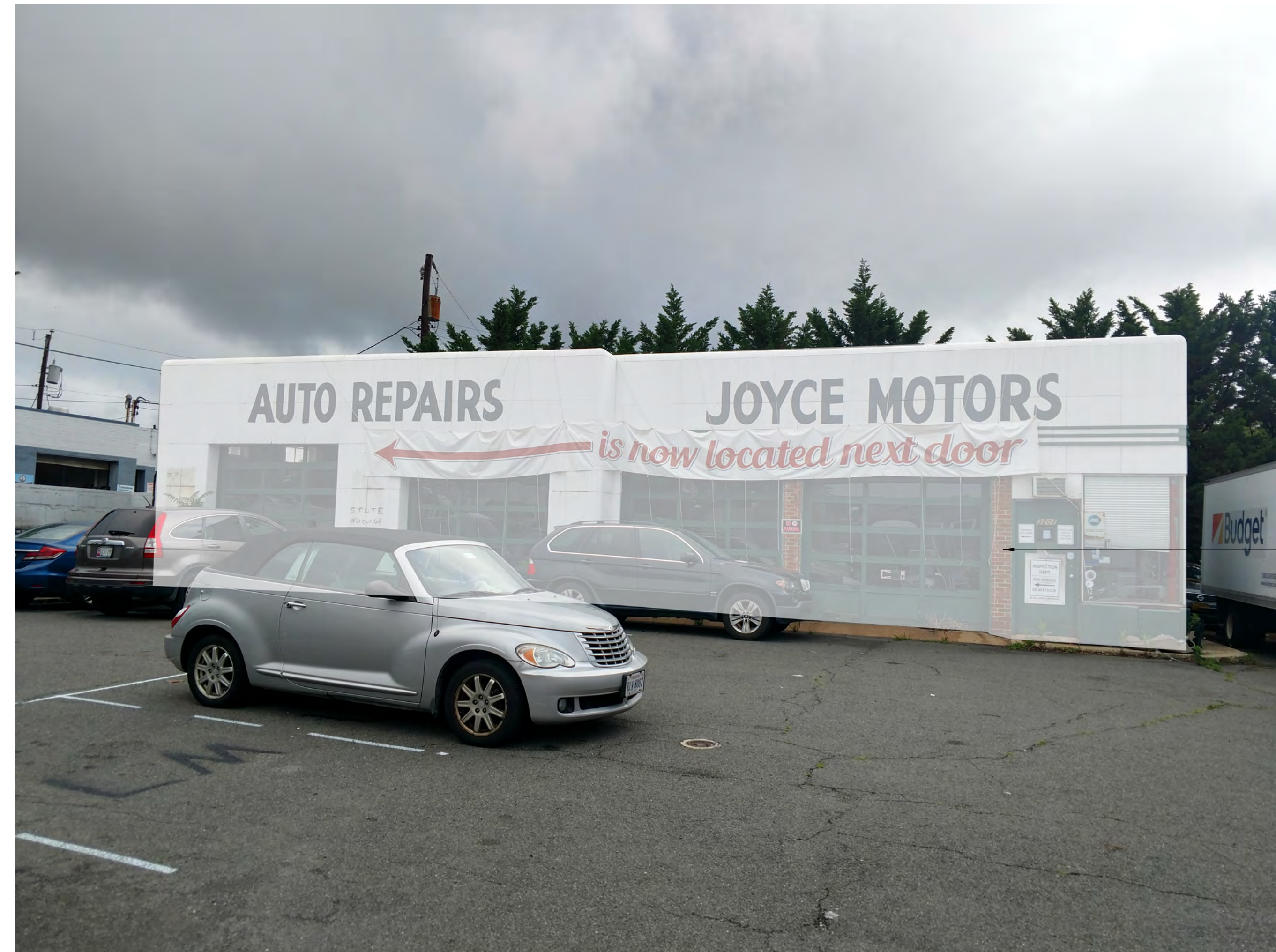
JOYCE MOTORS SOUTH FACADE
