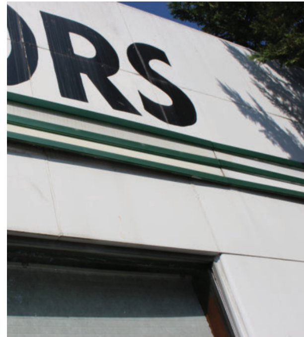
Figure 003 Detail of porcelain enamel panels. EHT Traceries, December 2018.
