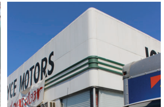
Figure 018 Curved edges at corner and speedlines. EHT Traceries, August 2019.
