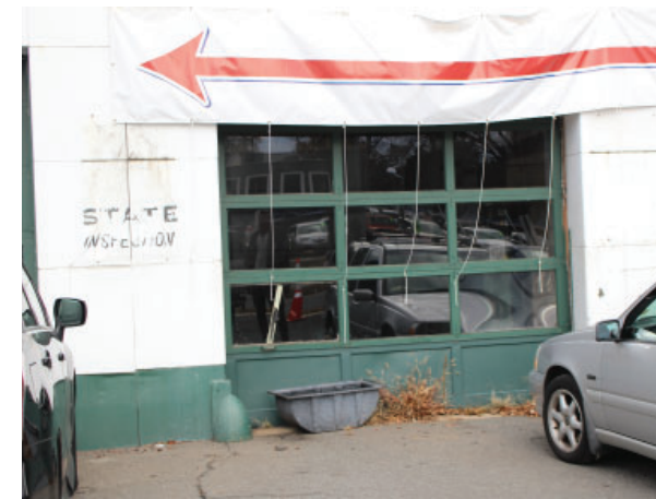
Figure 015 Detail of garage bay doors. EHT Traceries, August 2019.
