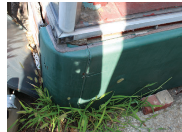
Figure 017 Detail of green porcelain enamel panels with rounded corner. EHT Traceries, August 2019.
