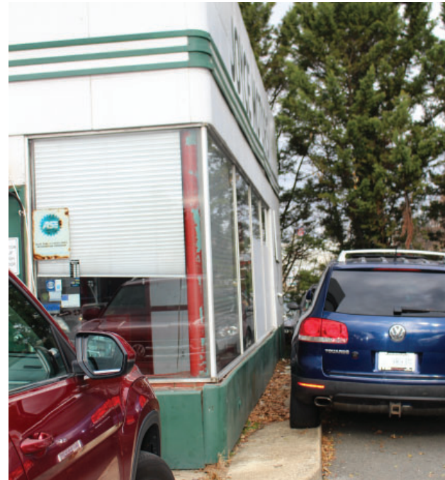
Figure 004 Detail of structural glass walls. EHT Traceries, December 2018.
