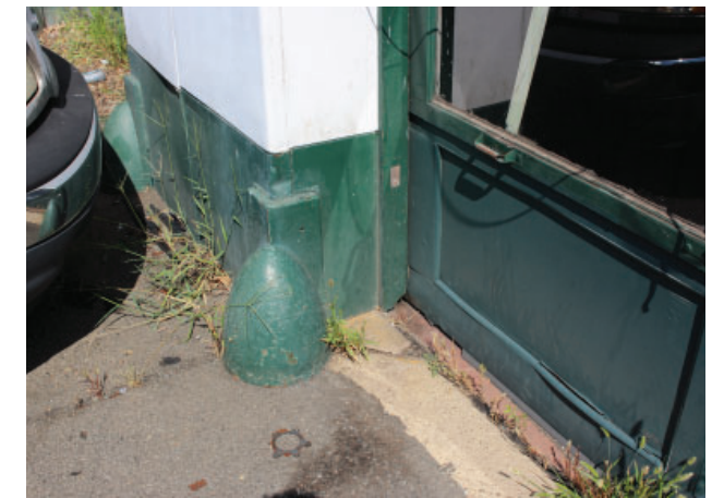
Figure 016 Corner bumper guards at garage bay entrance. EHT Traceries, August 2019.
