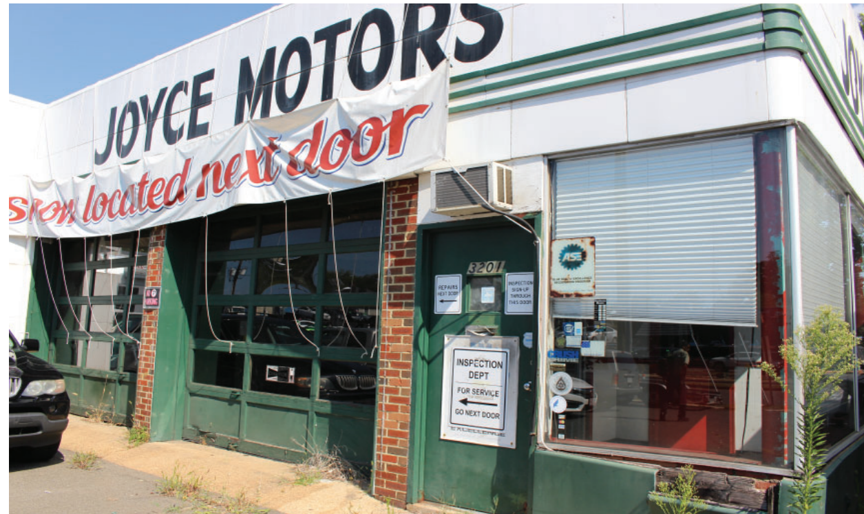
Figure 002 Joyce Motors, primary elevation. EHT Traceries, August 2019.
