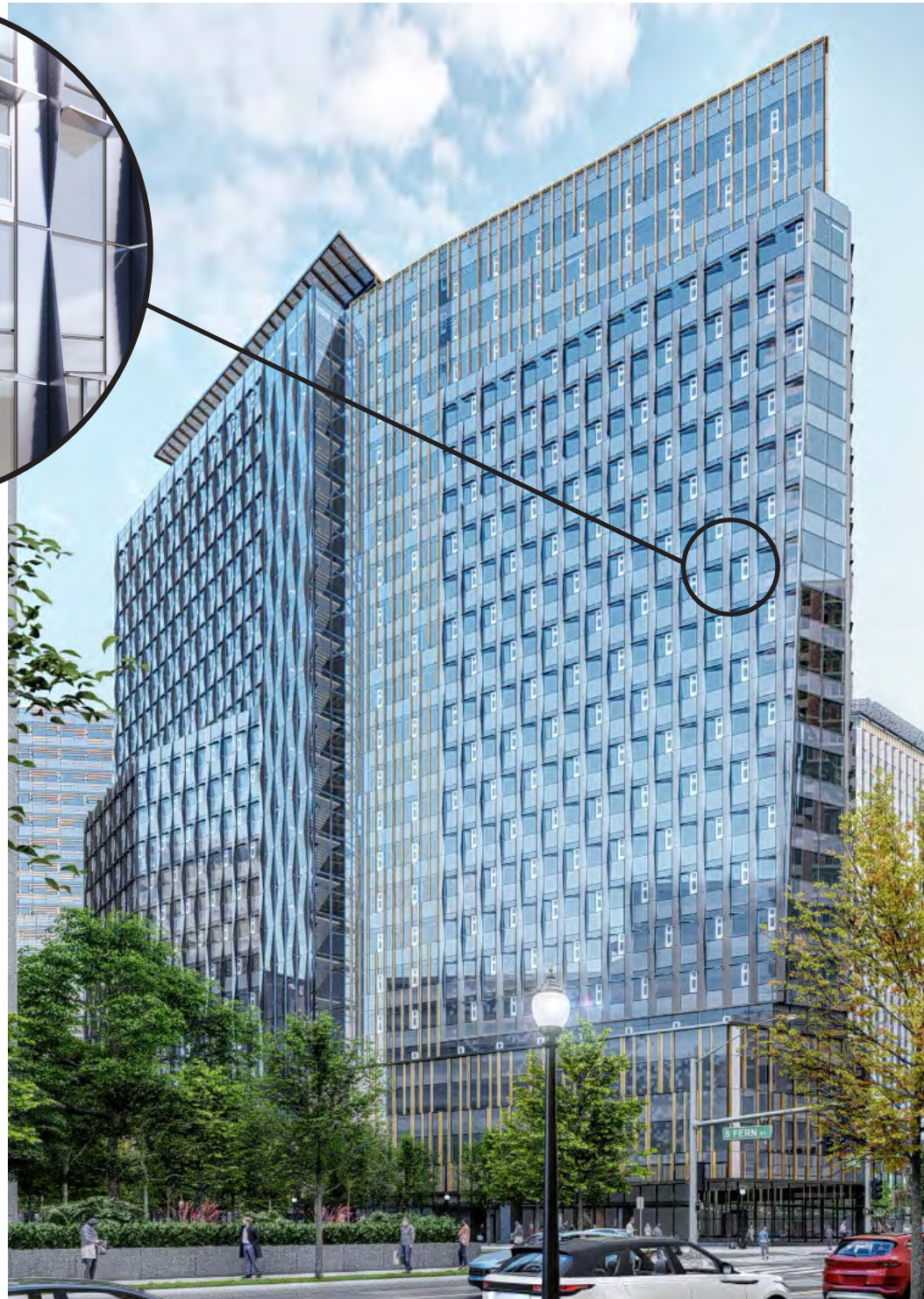
FINS TAILORED TO SOLAR DIRECTIONS FOR VISUAL COMFORT & MAXIMIZED COOLING EFFECT
