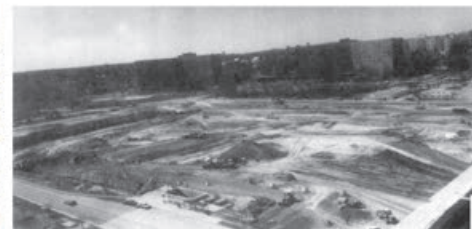
Construction of Pentagon City Mall
