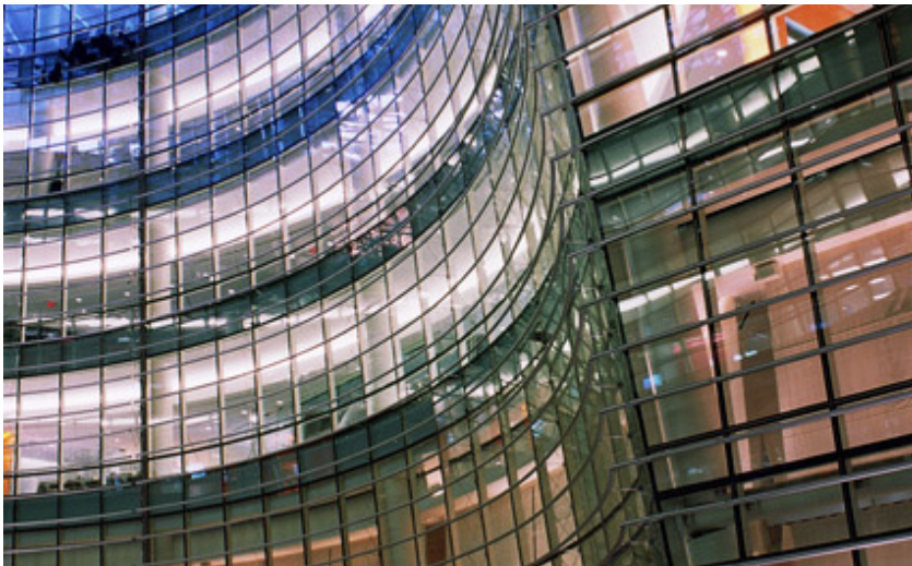
GLASS CURTAIN WALL
