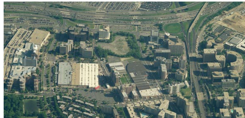
Existing Conditions Around Site
