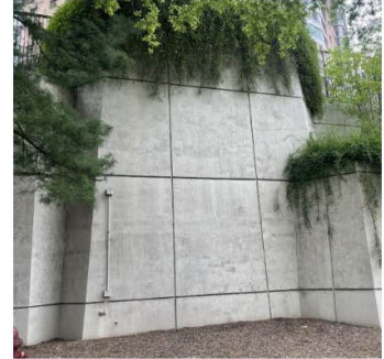
D SIDEWALK: COMPRESSED SPACE & HIGH RETAINING WALLS
