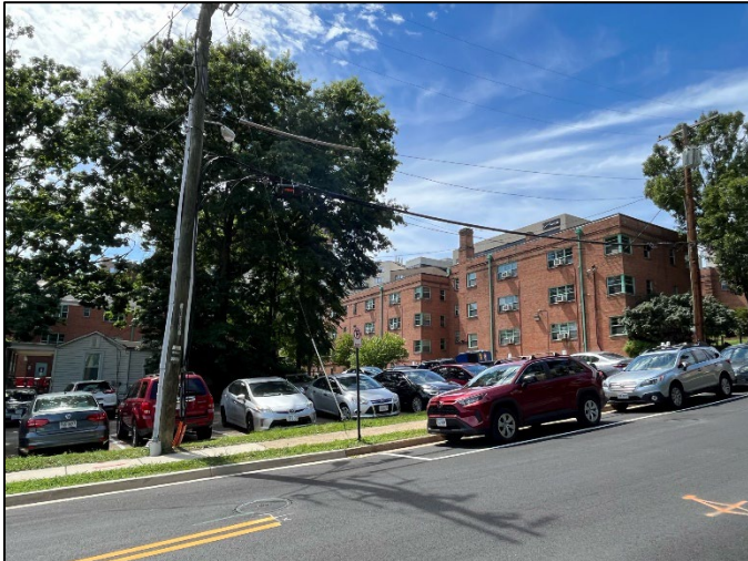
Figure 9. View of New Development Site from North Troy Street
